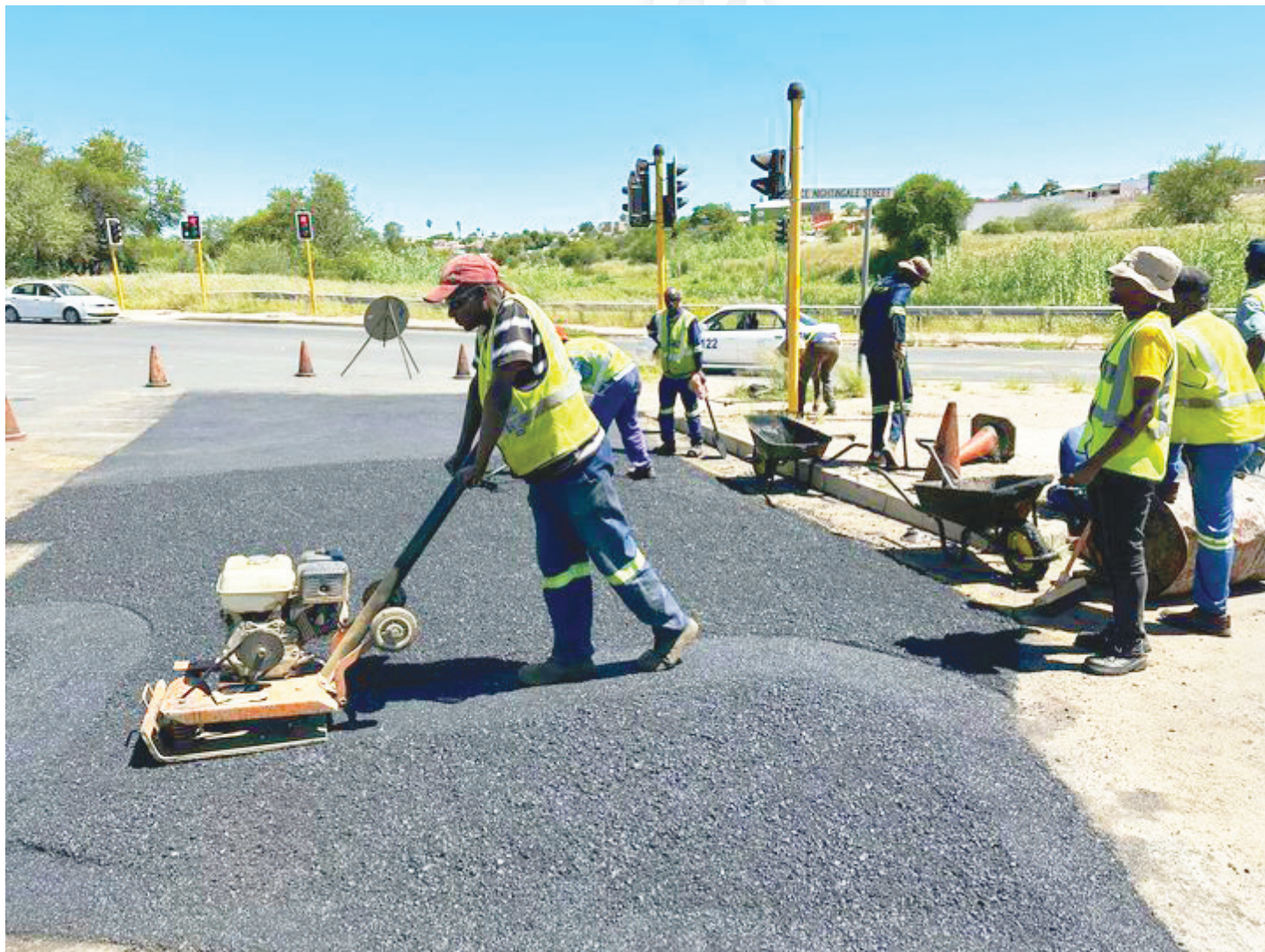
The Ujama Road Construction Company working on the corner of Shanghai and Florence Nightingale Streets, fixing the rain-damaged road surface. This work is part of the road rehabilitation exercise currently underway around Windhoek.
