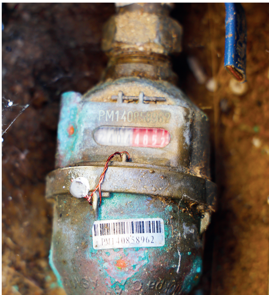
Municipal water meter showing the reading from left to right. Only the black numbers are recorded when taking the meter reading.
