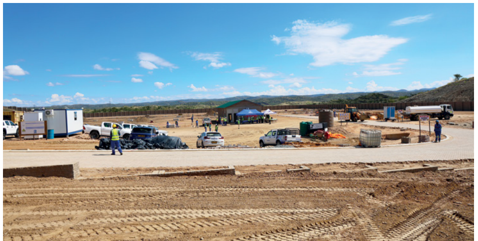
Cleared space for the Khomas Intake Substation
