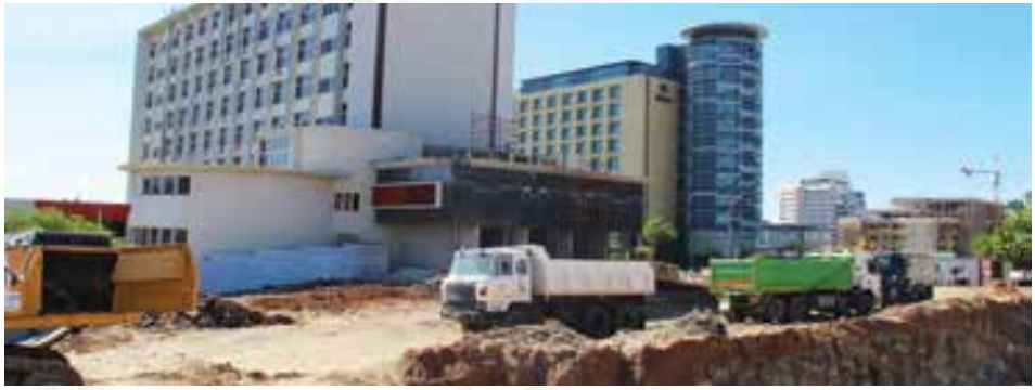
Construction work underway at the City of Windhoek Head office
